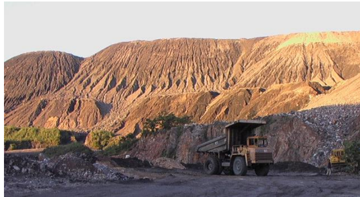
Figure 1: Erosion on waste rock dump slopes
