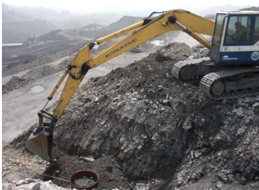
Figure 4: Trial pit for field testing
